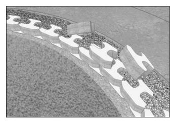
When building multiple courses on a curve, begin installation by placing a block in the middle of the curve and centering it on two blocks directly below it. Build the wall from the center block outward.
