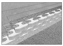
below it. Place core and drainage fill as in Step 4. Place the backfill material behind the drainage rock in maximum of 8" lifts and compact to 95% Standard Proctor. Repeat this process for each successive course.
