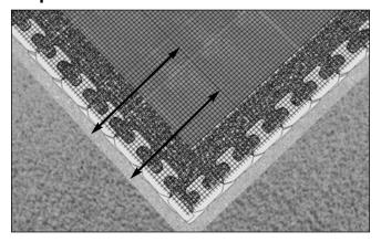
On an outside 90° corner, it is important that grid layers do not overlap at the corner. Place the first grid layer per plan at its design elevation and length.
