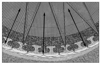
Overlapping layers of grid on a convex curve require a minimum of 3" of fill between them for proper anchorage. Repeat these steps for successive specified grid layers.
