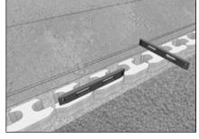
6" of base material in front and 6" behind the Base Block. Level each block, side-to-side, front-to-back and across three full blocks with a hand level. A rubber mallet may be used to level and align the blocks.
