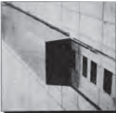
Figure 4.0 'C' Shaped Heater Duct
