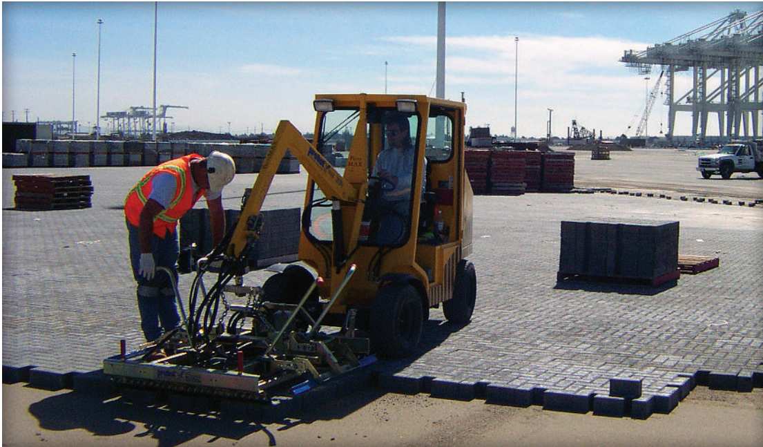
Figure 8. Mechanical installation equipment places concrete pavers rapidly.
